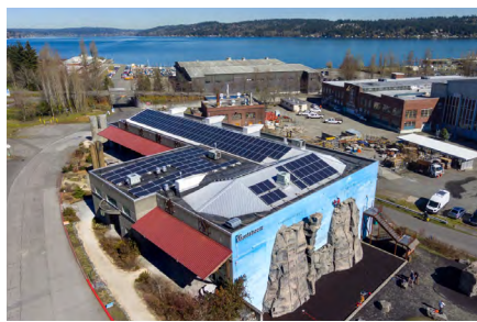
Our goal to achieve net zero carbon emissions from direct organizational impacts was codified into our strategic plan, with an initial focus on improving the buildings that support our programs and community.
